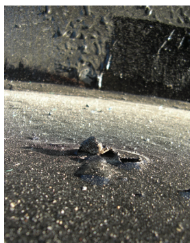
Fig 9: A blister in the liquid-applied waterproofing material that has been broken. If not rectified, this can be a problem spot which can compromise the waterproofing performance.
