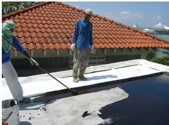
Fig 12: A primer being manually applied onto the receiving roof surface to provide a better bond for the pre-formed waterproofing membrane that will go on top.
