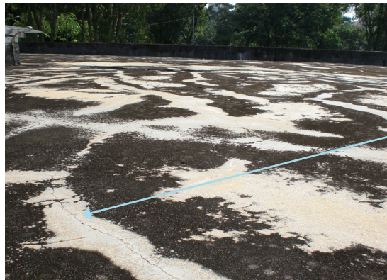
Fig 8: Cracks on an existing concrete roof
