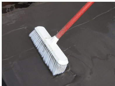
Fig 2: Liquid-applied waterproofing material can be applied through the use of a brush, roller, spreader or spraying device.
