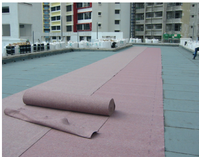
Fig 18: In less complicated site conditions, the protection mat can also be used to cushion the underlying waterproofing layer from physical damages.
