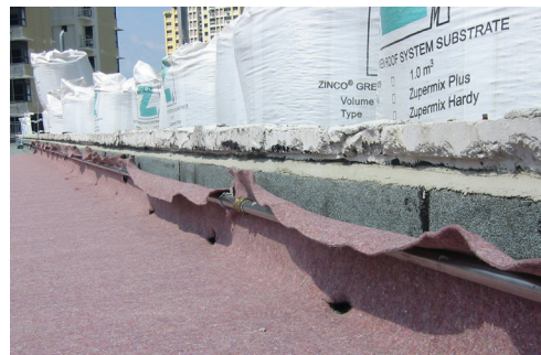
Fig 19: On horizontal and vertical surfaces, the protection mat can easily be laid over to protect the underlying waterproofing layer.
