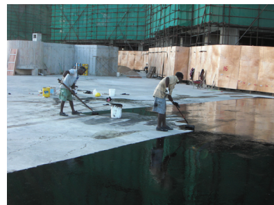
Fig 3: Liquid-applied waterproofing material is manually applied through the use of rollers.
